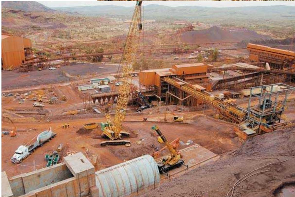
Two TechSpan arch tunnels have been built on the site of Mount Tom Price: one houses a receiving conveyor (see photo above) and the other an emergency exit.
