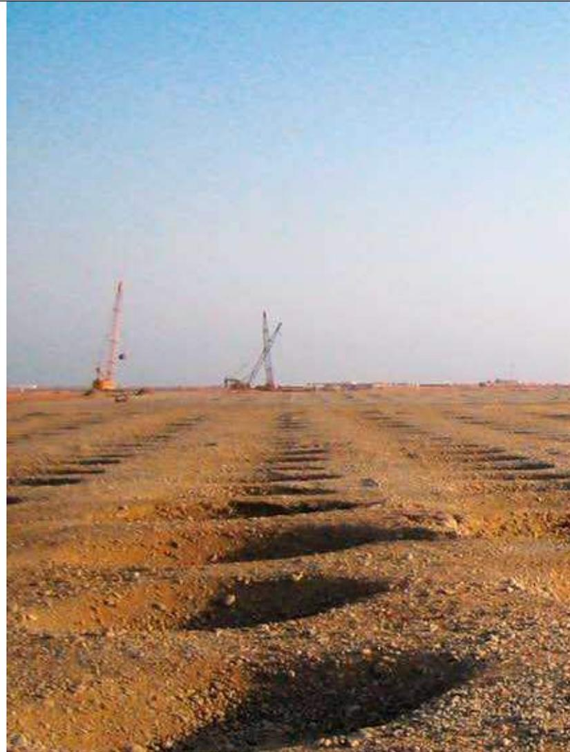
the work. "The presence of a shallow water table and the soil type meant that work also had to take place in various phases, representing up to five work phases for the same area, leaving the soil to rest between each phase," explains Arnaud Meltz, project technical lead for Ménard.
