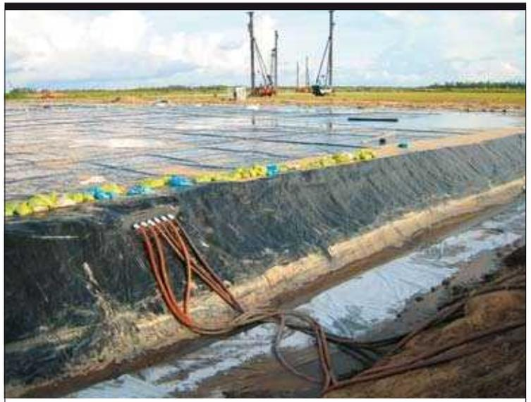
**2005** In southern Vietnam, the Cai Mau power station was to be built on 161 ha on the banks of the Cai Tau river. 240,000 m<sup>2</sup> of soil required consolidation, 90,000 m<sup>2</sup> of which had to be completed in under one year. To meet this deadline, Ménard divided the site into
