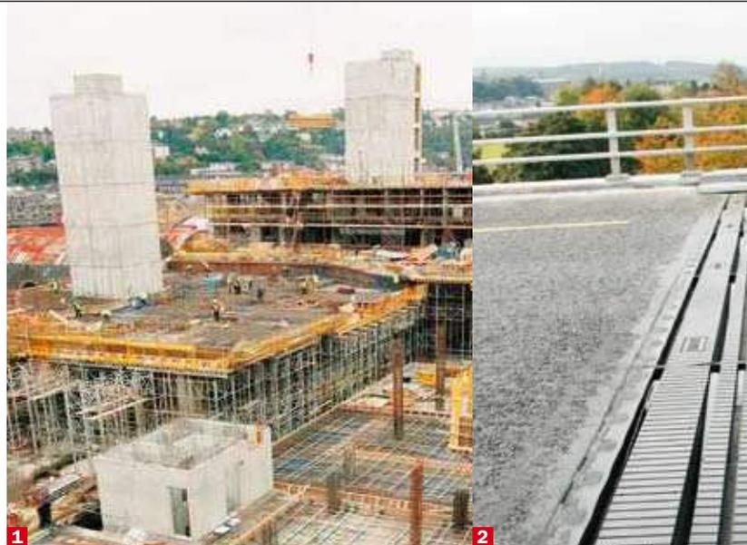
1. The Elysian complex project used a total of 33,000 m<sup>2</sup> of prestressed floors, using 300 tonnes of steel, and deployed a team of 12.
