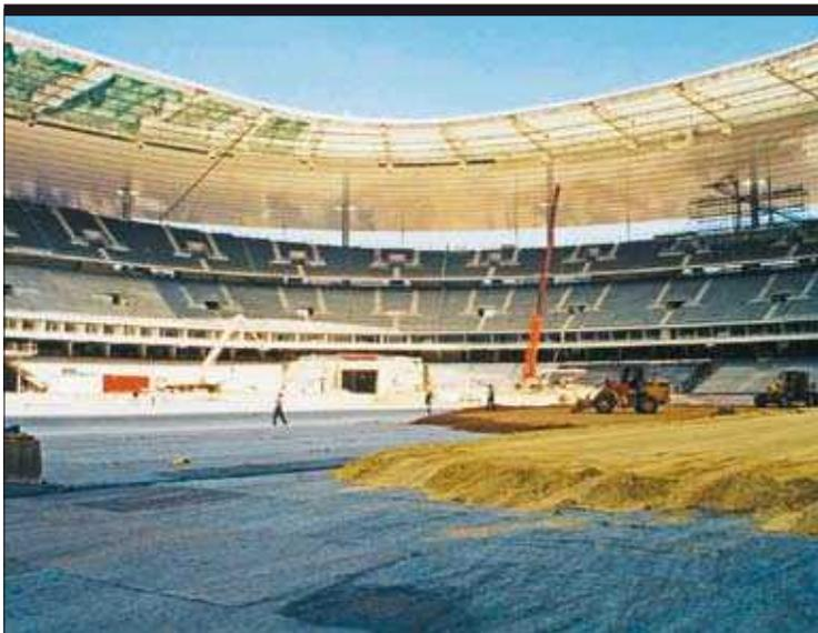
**1997** An alternate of the Menard Vacuum process, a venting system based on the use of drains and pumps and a waterproof membrane was installed under the Stade De France (St-Denis, France) to treat the gas fumes coming from
