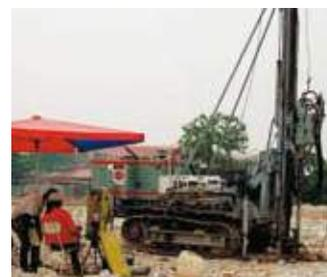
**Malaysia.** As a preliminary stage to constructing the east coast motorway linking the cities of Kuantan (in the South) and Kuala Trengganu (in the North), Menard Geosystems carried out soil improvement work over a 130,000 m<sup>2</sup> area. Two techniques were used: dynamic compacting and vertical drains
