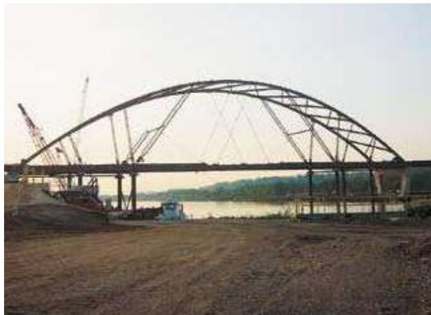
**United States.** On the borders of West Virginia and Ohio, Freyssinet has completed the installation of the stay cables on the Blennerhasset Island Bridge, an arch bridge crossing the Ohio very near Parkersburg. The structure consists of a prestressed mixed deck suspended by two planes of
